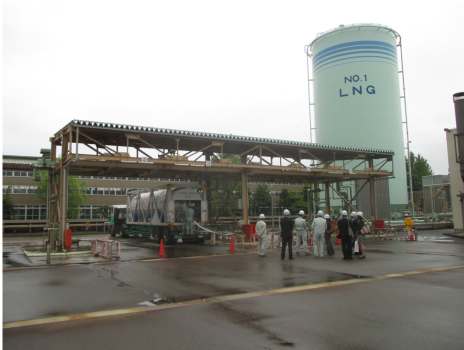
Photo 8: Unloading LNG Containers at Distributorship in Kanazawa: photo Richard D. Stewart
