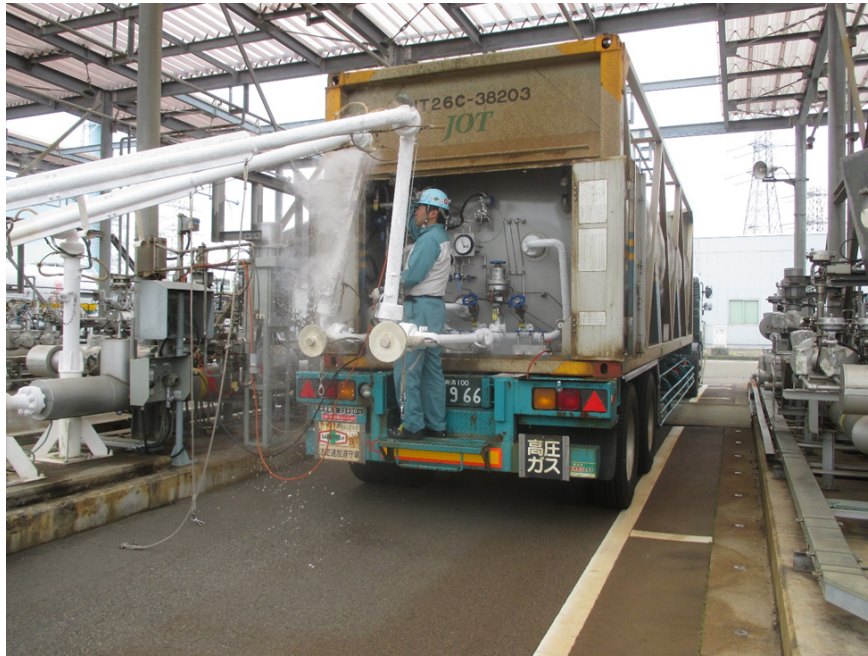
Photo 4: Loading LNG into container at JAPEX Niigata facility. Photo by Richard D. Stewart
