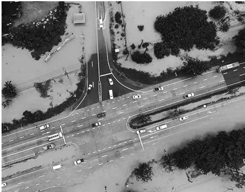
Figure 1 Inadequate Drainage Structure on Road
